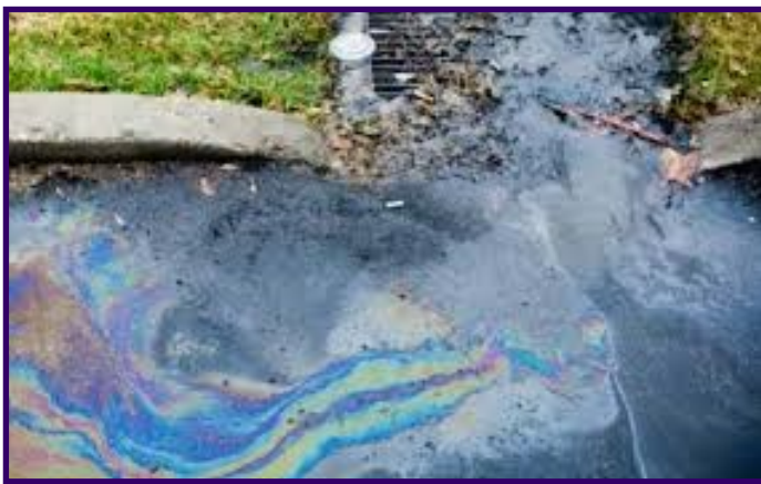
Oily substances are a sure sign that an illicit discharge has occurred.
