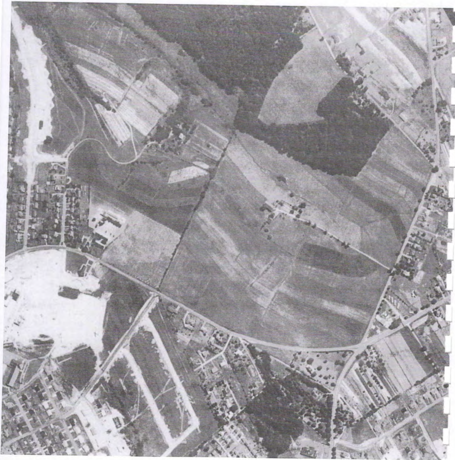
1957 AERIAL WITH YORK SUBURBAN HS UNDER CONSTRUCTION
